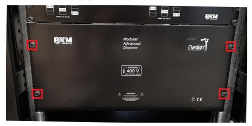
Then remove the cover of the copper bars.
