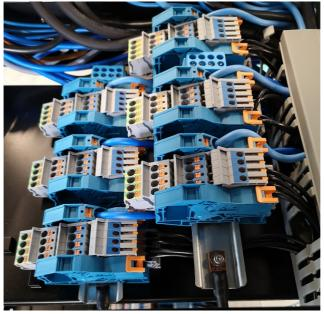
**NOTE!** The phase, neutral and ground wires of one receiver must be connected to the same terminal group.
