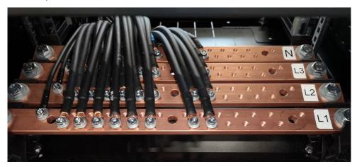
The busbars have connection holes for an M10 screw, which must be tightened with a torque wrench with a force of 50Nm. The cables must be equipped with cable lugs for an M10 screw.
